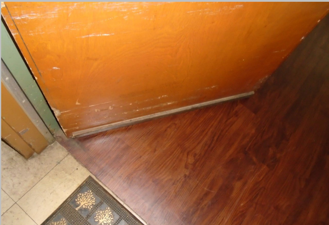
UNIT DOOR CONDITION
