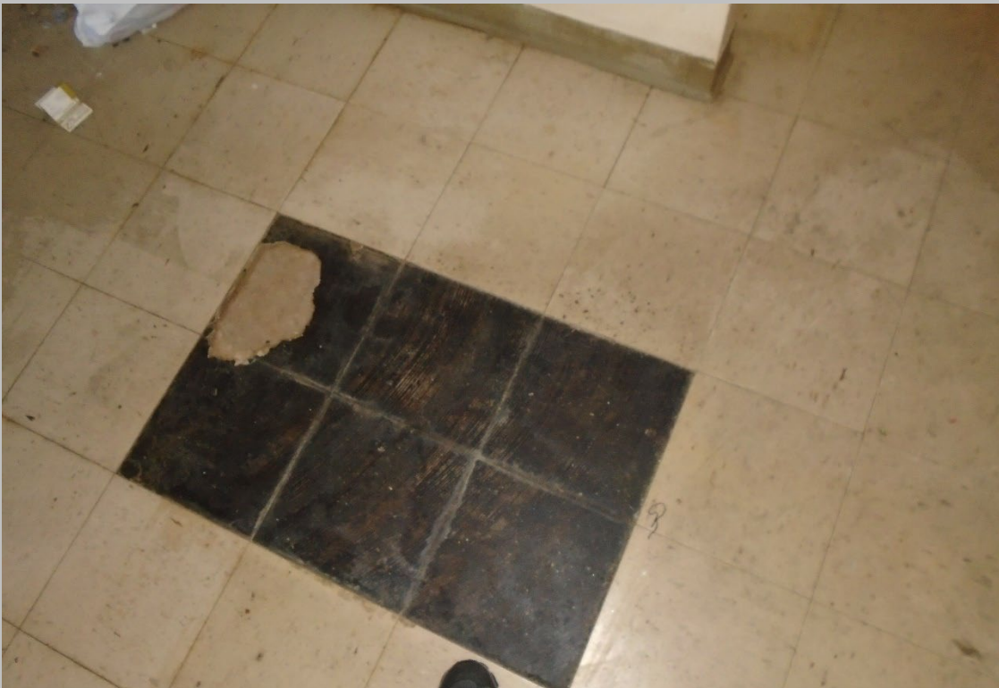
UNIT FLOOR CONDITION
