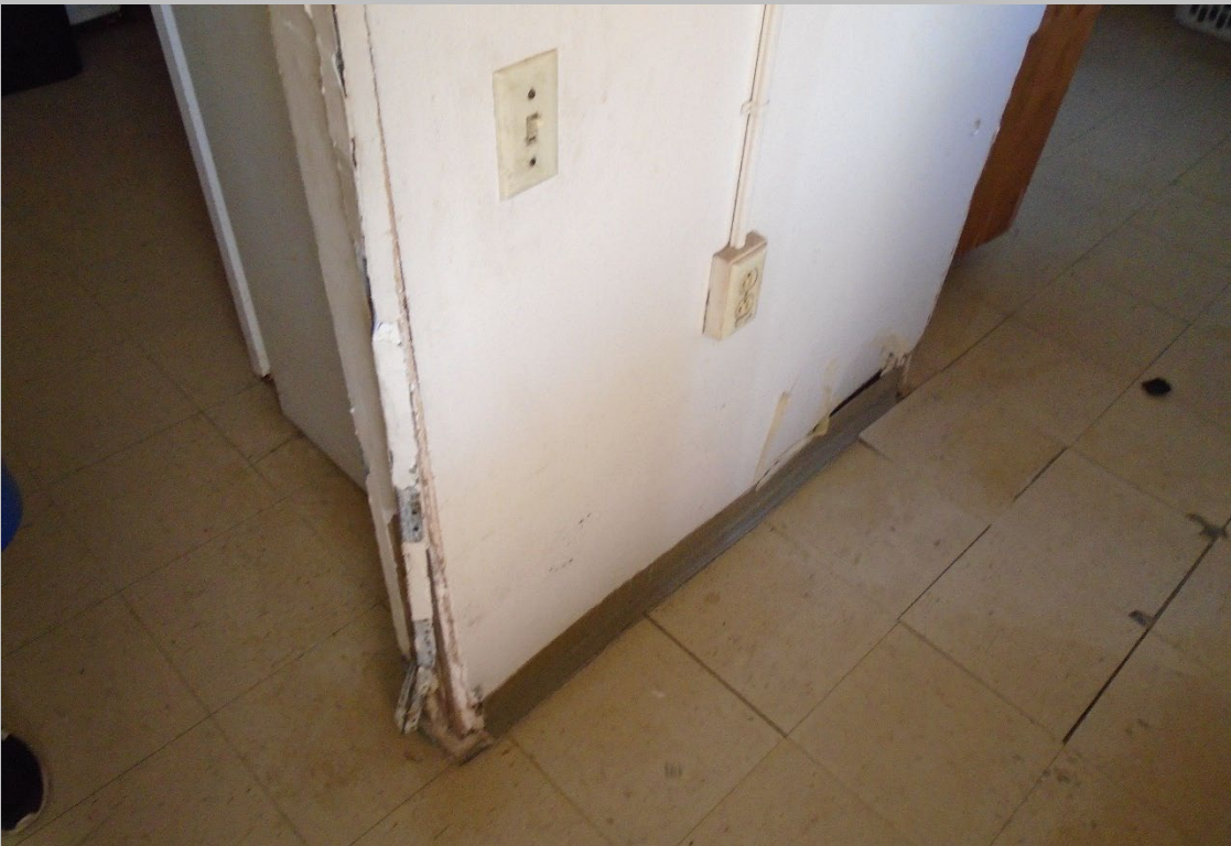
ISOLATED DRYWALL NEEDS
