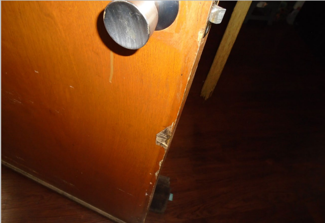
UNIT DOOR CONDITION
