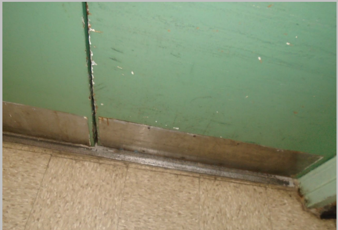
INTERIOR DOOR CONDITION
