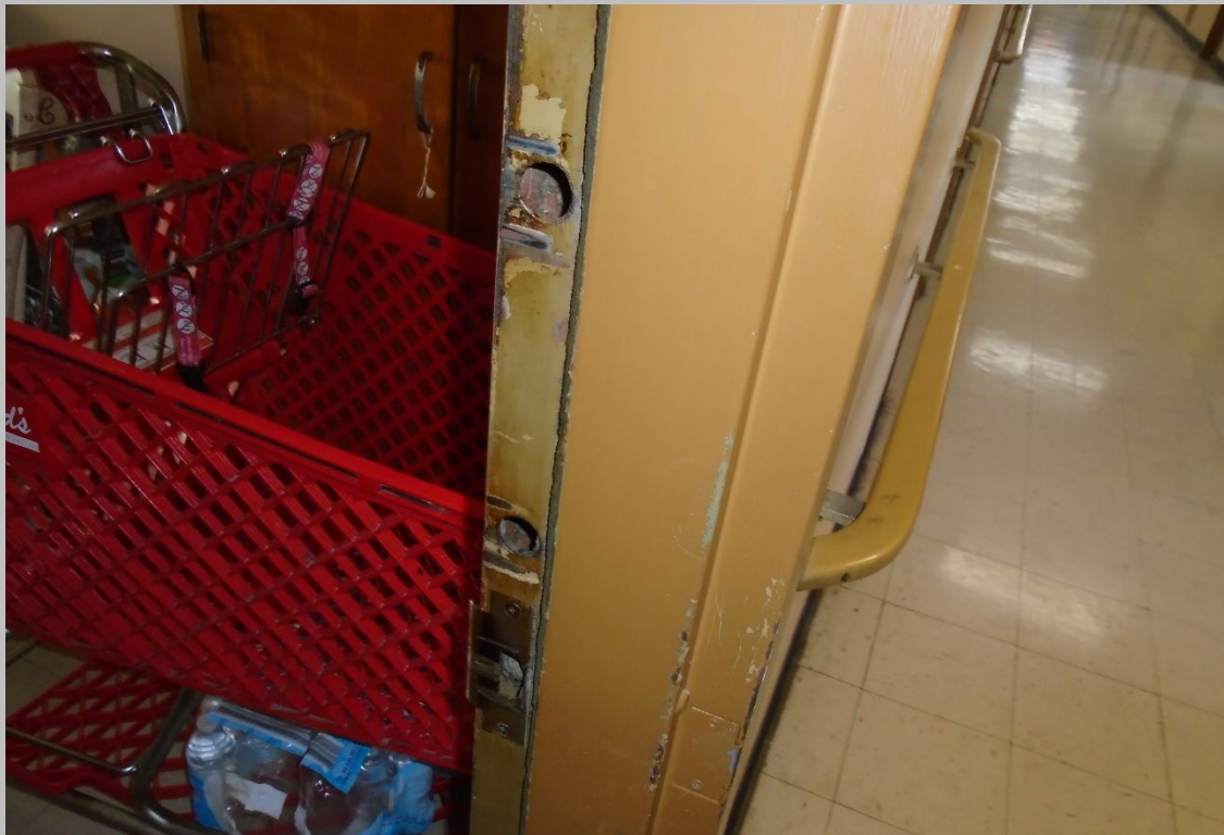
UNIT DOOR CONDITION
