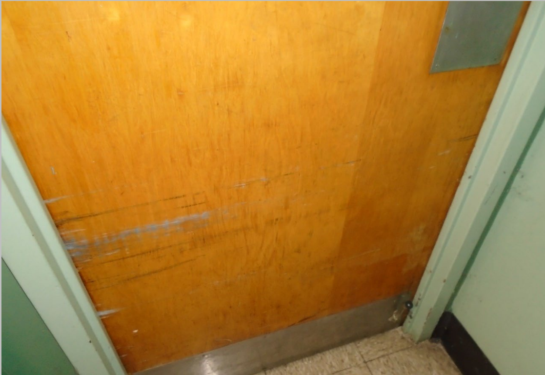
INTERIOR DOOR CONDITION
