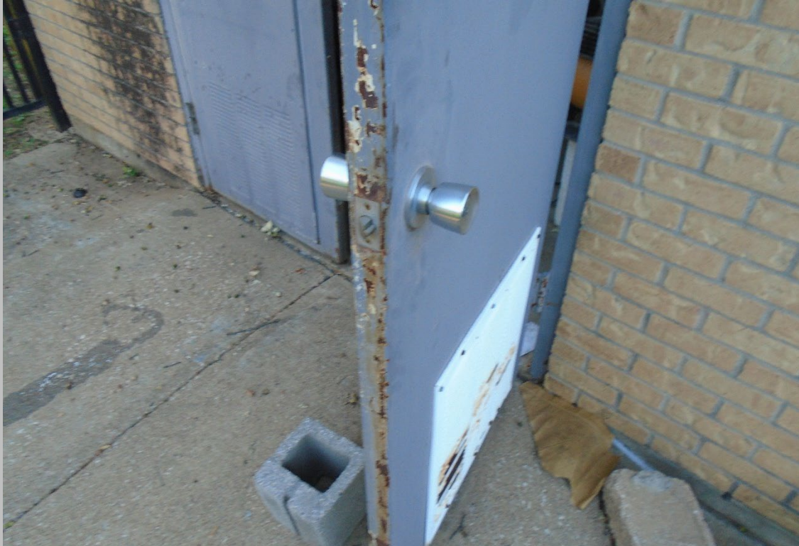
EXTERIOR DOOR CONDITION
