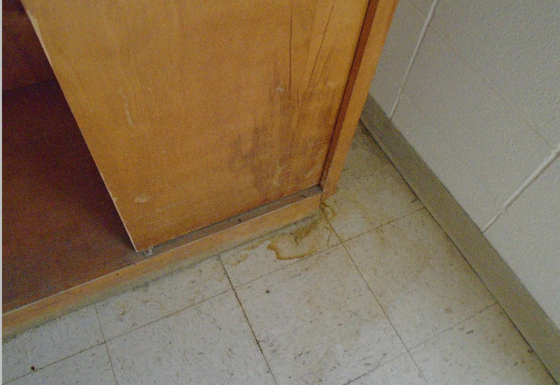
UNIT FLOOR CONDITION
