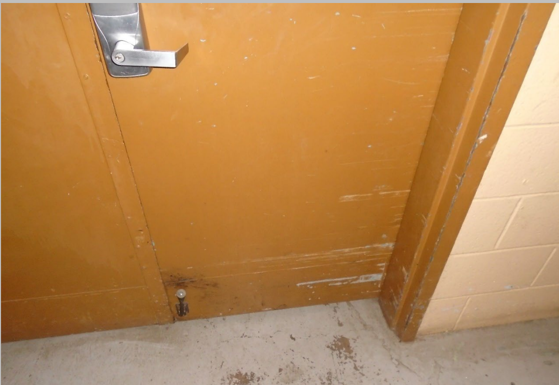
INTERIOR DOOR CONDITION
