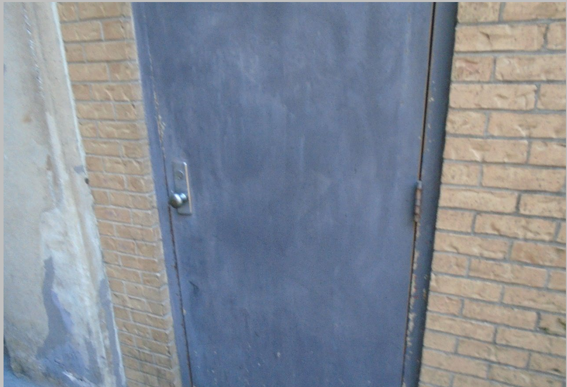
EXTERIOR DOOR CONDITION
